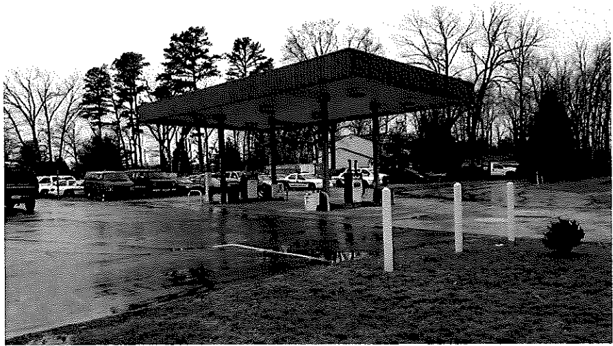
View 1: Showing Fuel Dispensing Station
